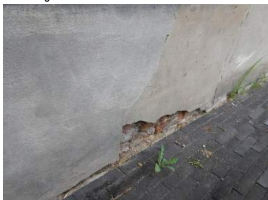
loskomende cementering
