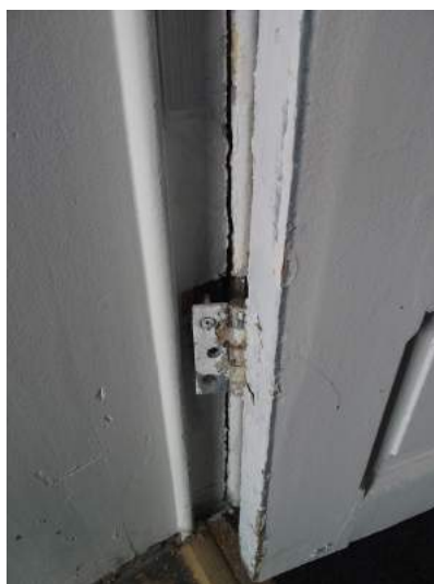
Defect scharnier
